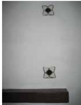
Air ducts, Spain
