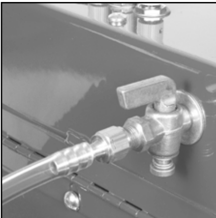
Fig 25 - Water control inlet valve with valve in the open position
